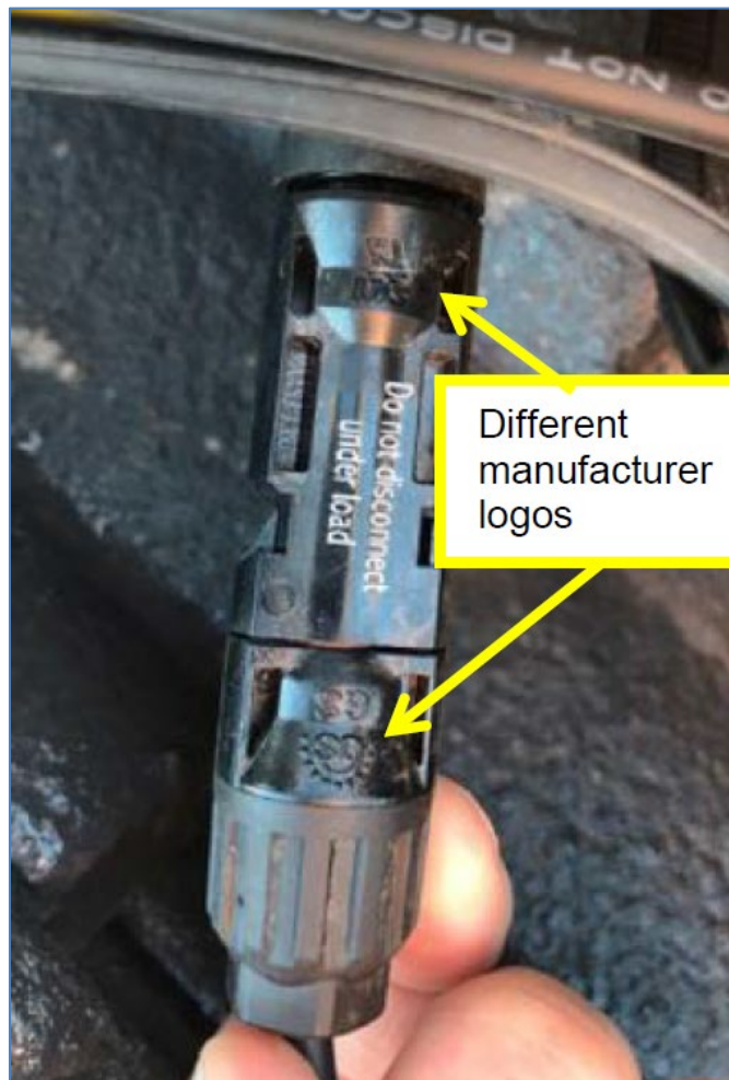
Example of d.c. connector showing mismatching manufacturer logos
