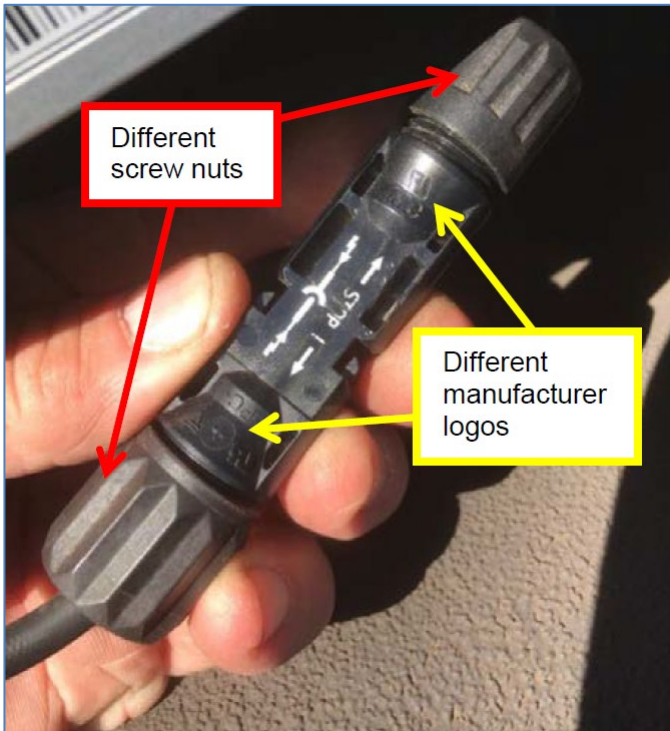
Example of d.c. connectors with mismatching screw nuts, manufacturer logos and body mouldings
