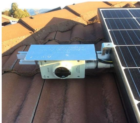
Image 1 & 2 Non-compliant - Shroud does not provide adequate protection from direct sunlight
