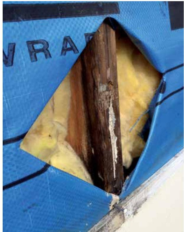
Fig. 35. Vapour impermeable building wrap traps water vapour in walls
