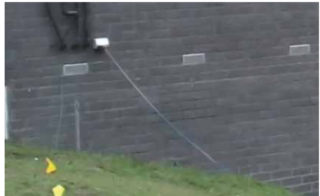
Fig. 43. Evenly spaced subfloor vents in masonry wall
