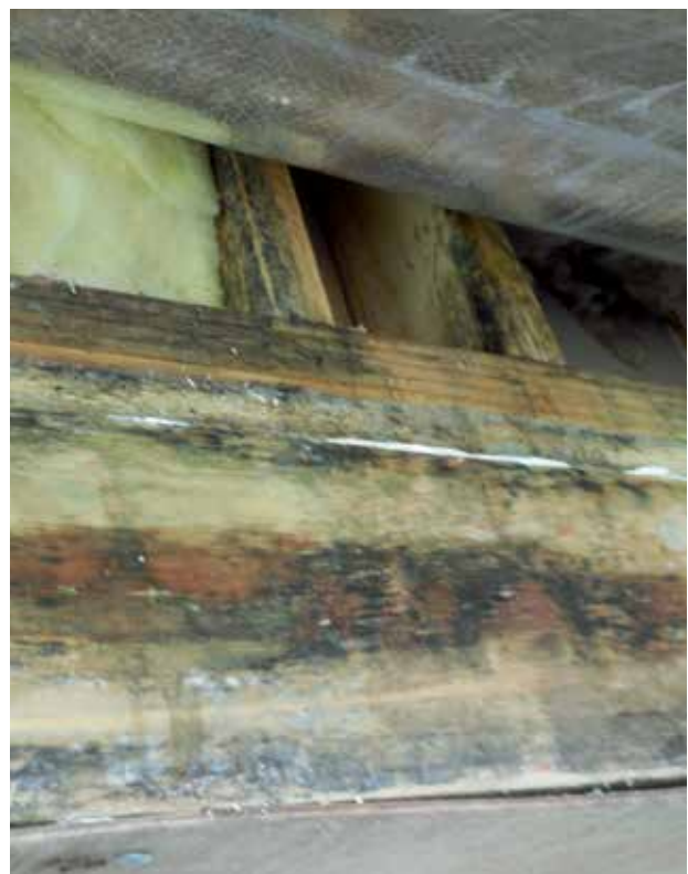
Fig. 36. Mould and rot in wall structure caused by air leakage
