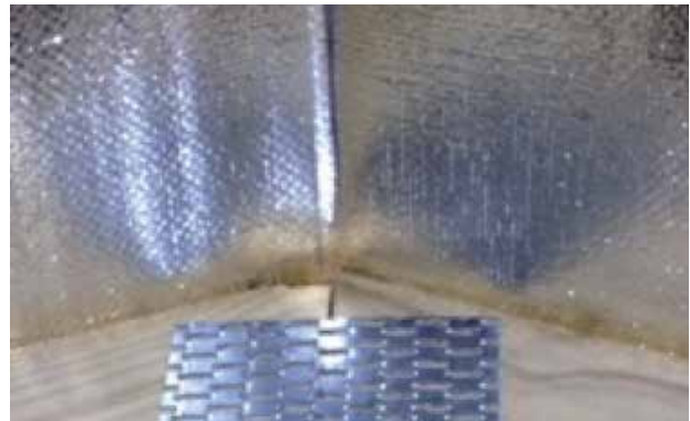
Fig. 13. Continuous gap in sarking along ridge
