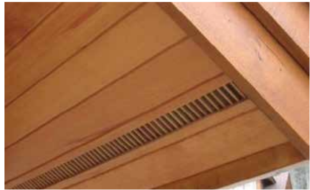
Fig. 12. Continuous eave vent
