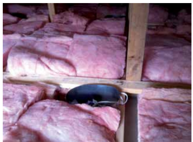
Fig. 8. Thermal bridging due to lack of insulation around downlight
