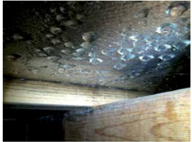
Fig. 6. Thermal bridging between roofing and sarking
