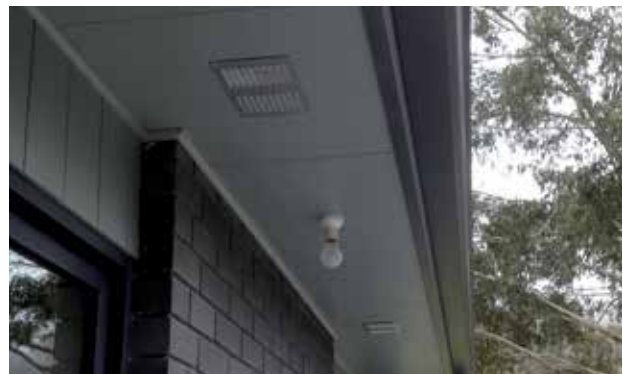
Fig. 14. Regularly spaced eave vent
