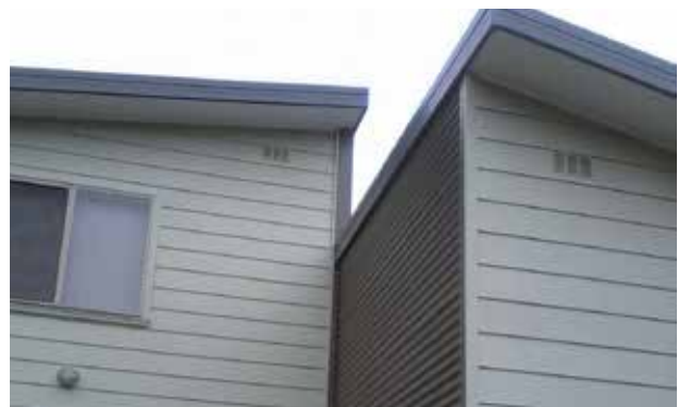
Fig. 15. Regularly spaced gable or parapet vents
