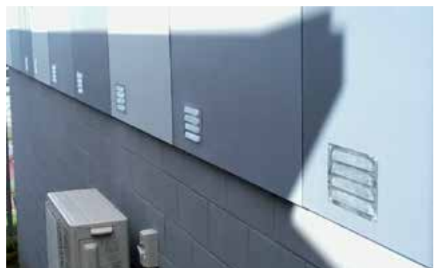
Fig. 44. Subfloor vents in clad wall
