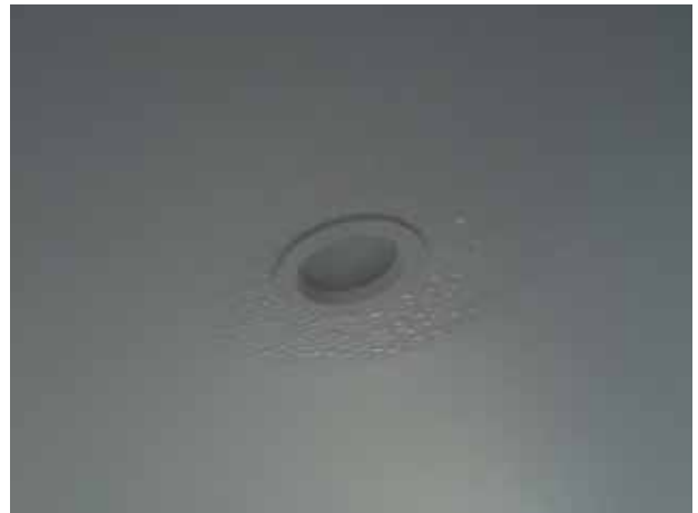
Fig. 7. Thermal bridging around downlight
